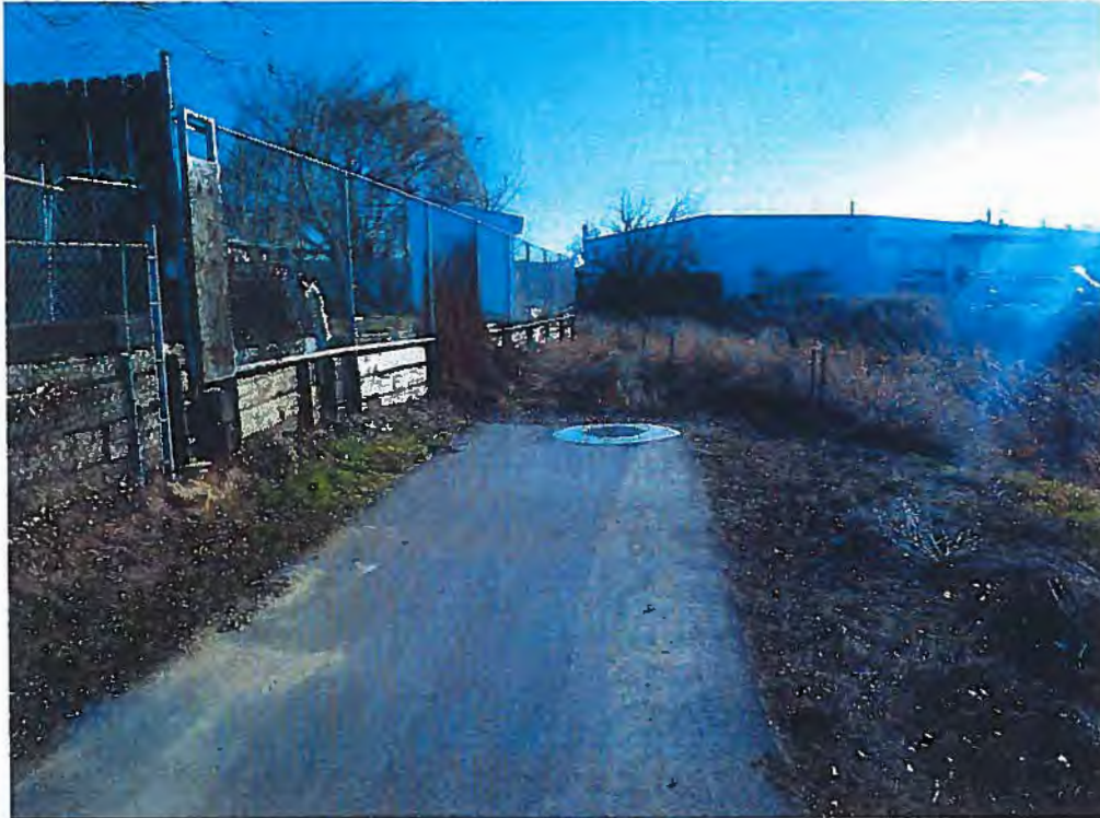
Point of west connection to existing pathway.
