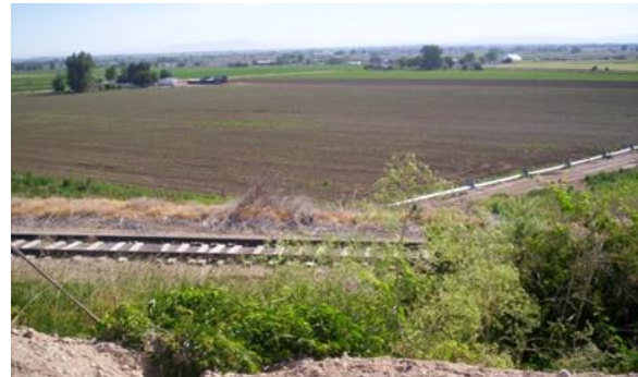
View of RR Tracks from Antrim Drive, looking northeast
