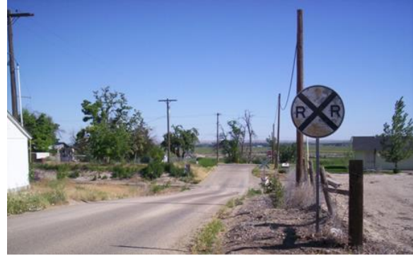
Academy Road RR Crossing, looking north towards Peckham Road
