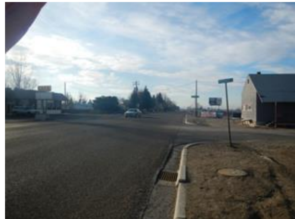
SH 19/Friends Road Intersection
